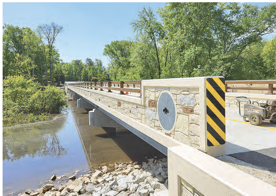
The bike trail bridge over Dogue Creek is nearly complete.
