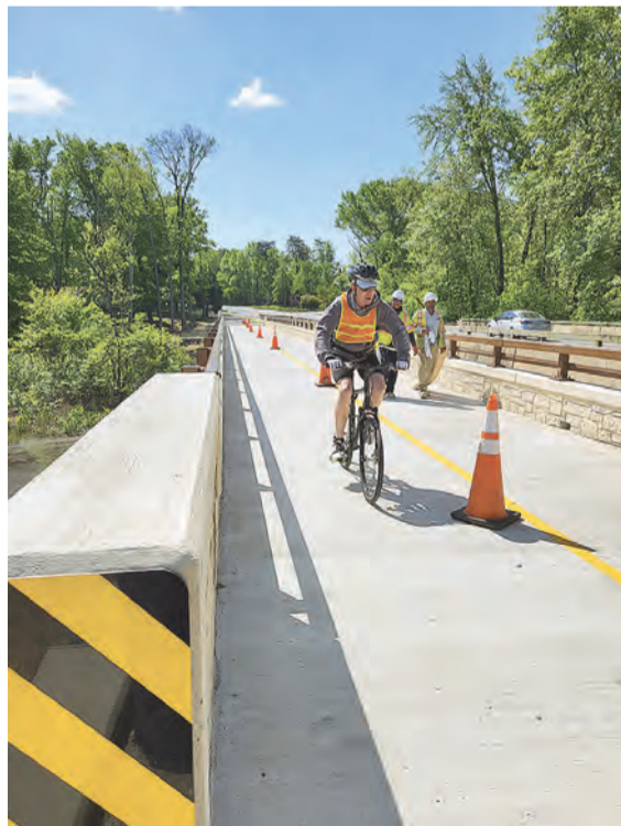
This new bridge over Dogue Creek is a connector to the Mount Vernon Trail on the southern end.
